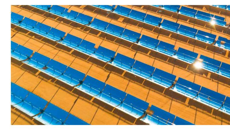
When solar energy for electricity generation is discussed, photovoltaic systems most often come to mind. However, concentrated solar power systems are gaining popularity as an interesting alternative. In these type of power plants, collector systems concentrate sunlight and collect it on an absorber pipe. A heat transfer fluid in these absorbers or receivers transports the energy to a turbine which is connected to an electrical power generator.
