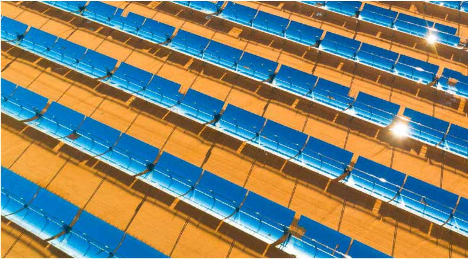
When solar energy for electricity generation is discussed, photovoltaic systems most often come to mind. However, concentrated solar power systems are gaining popularity as an interesting alternative. In these type of power plants, collector systems concentrate sunlight and collect it on an absorber pipe. A heat transfer fluid in these absorbers or receivers transports the energy to a turbine which is connected to an electrical power generator.
